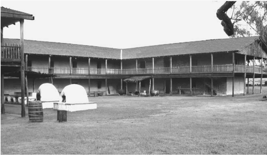
Figure 2 Remaining three-quarters of quadrangle of Petaluma Adobe, Petaluma Adobe State Historic Park, California. Photo: Stephen Silliman
