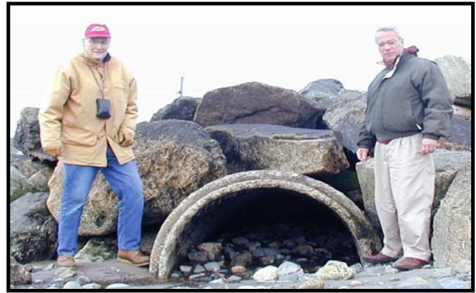
This 48-inch culvert was providing inadequate tidal flow to over 100 acres of salt marsh at Little River, Rye, NH. Photo by NHCP
