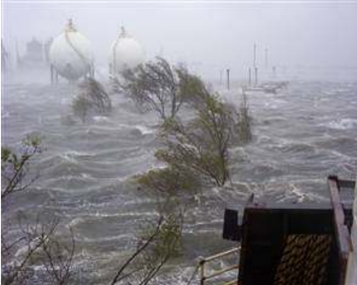
Figure 3: Storm Surge and Flooding Post-Katrina at Petrochemical Facility
